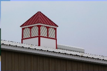
STANDING SEAM ROOF
